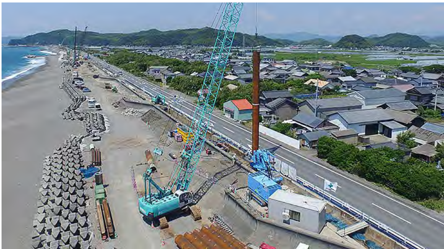
“Implant Levee” currently under construction along the Kochi coast (Tobara site)
