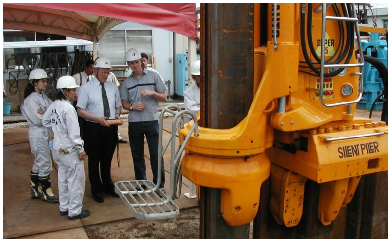
Fig. 1. The Cambridge team pressing-in piles: Gulin Yetginer, Malcolm Bolton and David White take turns to operate a Silent Piler under the watchful eye of Kayoko Yamamoto at Giken's Takasu facility in July 2001.
