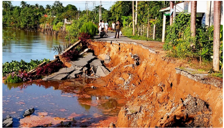
Fig. 2. Riverbank erosion in Dong Thap province of Mekong River Delta
