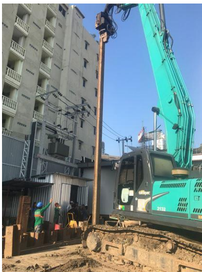
Photo 1 Vibro hammer technique
