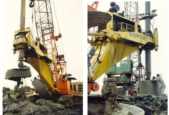
Photo 2. Photo of wet process bored pile
