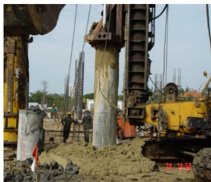
Photo 1. Photo of augering in sand layer
