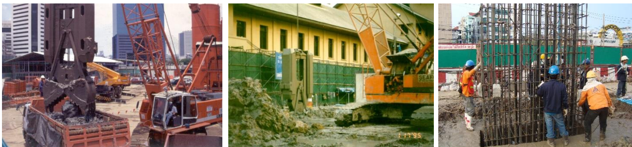
Photo 3. Photo during constructing barrette
