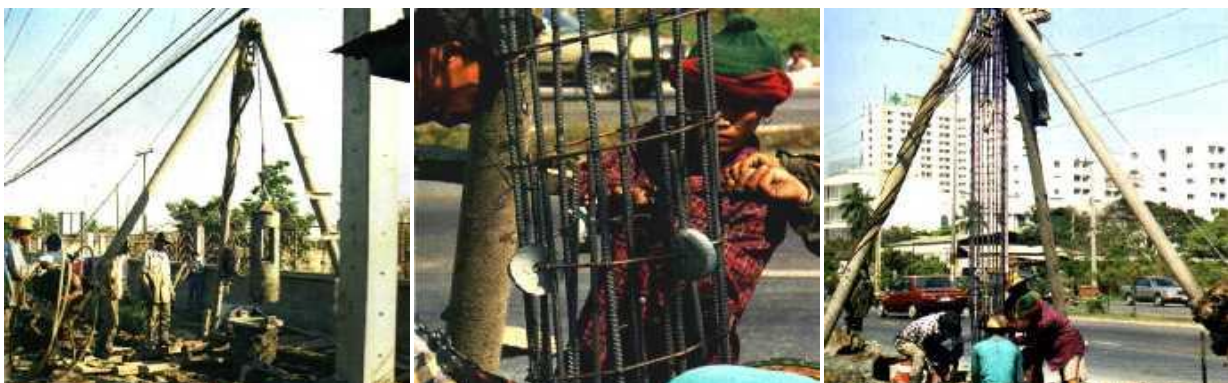
Photo 4. The schematic technique of dry process bored pile (continued)
