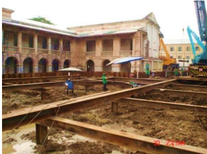
Photo 2 Sheet pile was driven around existing palace
