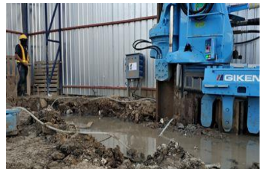
Photo 5 Sheet pile alignment and site fence
