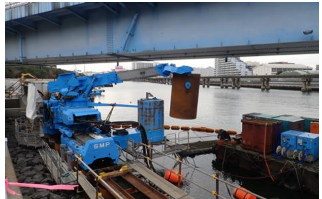
Photo 4. Low overhead type Piler with Y-jibu attachment
