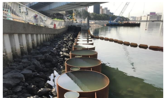
Photo 7. Completion of Press-in operation
