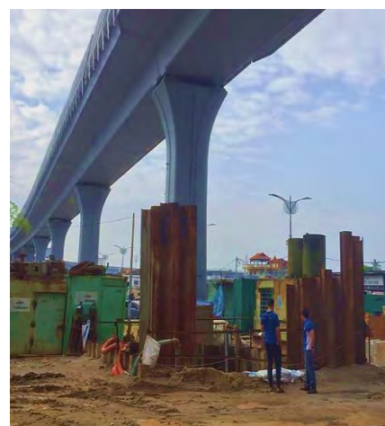
Fig. 4. Sheet pile installation under MRT Line
