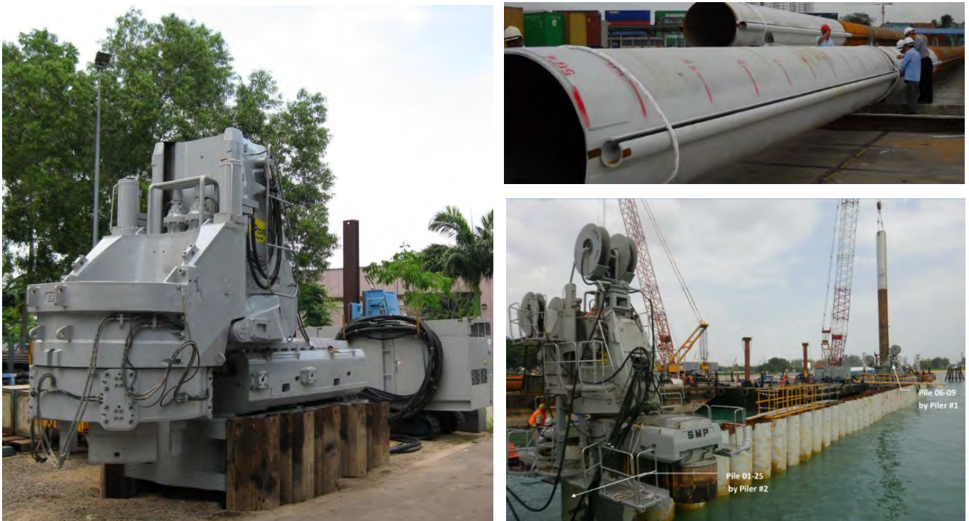
Figs. 6. GIKEN Kokan Piler & Tubular Sheet Piles
