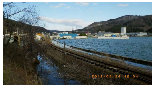
Fig. 4. Lowered ground level due to coseismic subsidence in Bansekiura near Sendai City
