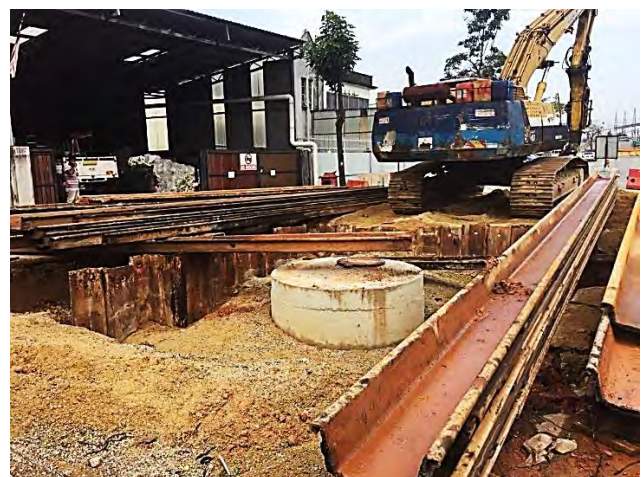
Fig. 2. Sheet pile work on construction site
