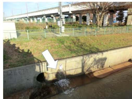
Fig. 16. Ongoing drainage and lowering of ground water level in Kuki City (photograph by Prof. Koseki)
