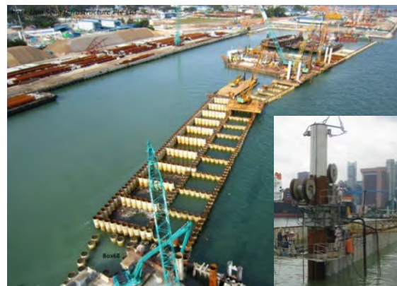
Fig. 4. Tubular Sheet Piles installed by Giken Kokan Piler
