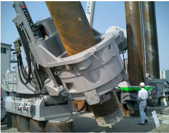
Figs. 7. Installation of Raker Pipe Pile with Rotational Cutting Bit using Gyro Piler
