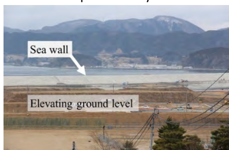
Fig. 23. Ongoing reconstruction of Rikuzen-Takata City
