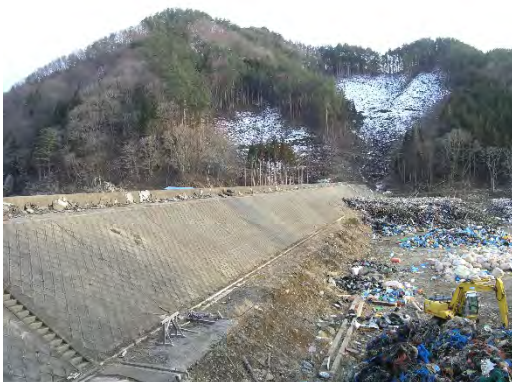
Fig. 7. Sea wall in Tohni-Hongo that was constructed prior the disaster in 2011
