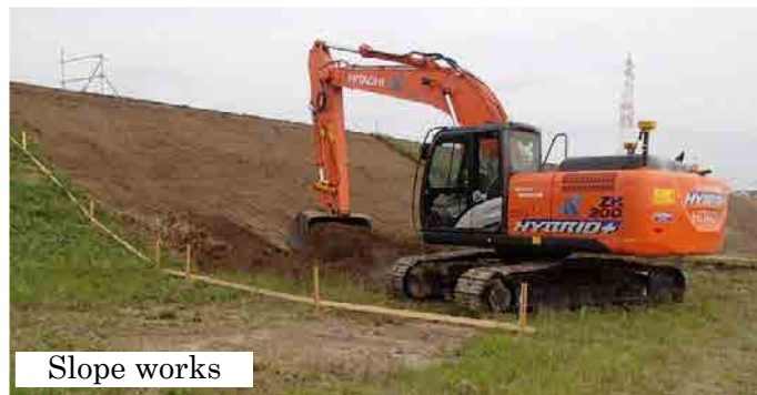
Figure 10 Typical works with hydraulic shovel
