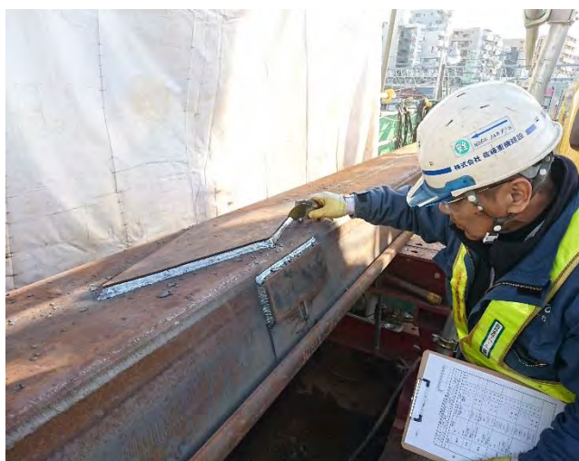
Picture7 Mr. Matsuzawa is checking lateral joints on the site
