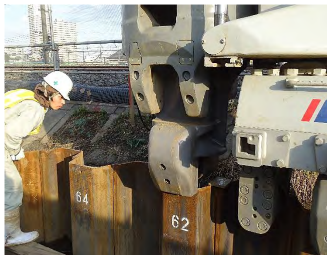
Picture8 Mr. Asano is operating the system of self-waling backward
