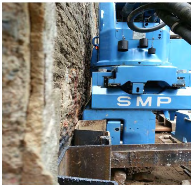
Figure 3 Zero clearance press-in method
