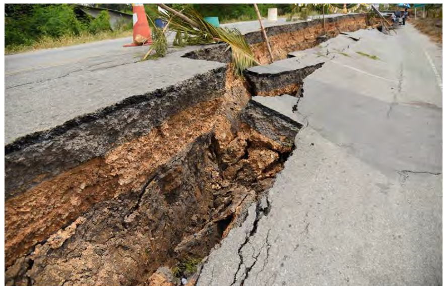
Photo 1 Road settlement alongside of irrigation area canal
