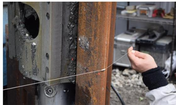
Photo 6 Checking sheet pile position with the Piler laser
