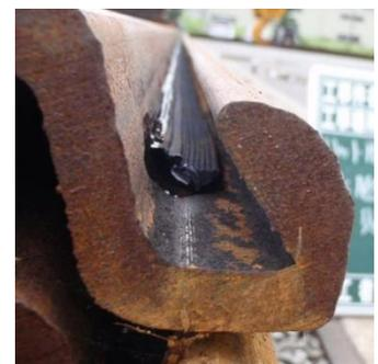
Photo 4 rubber water cut-off seal
