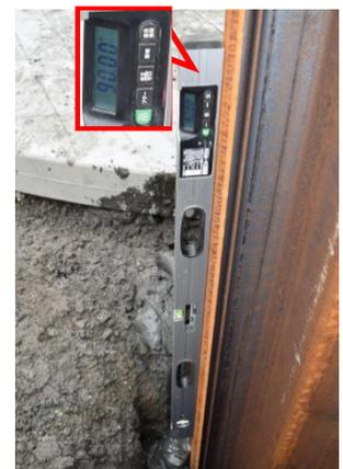
Photo 3 Checking distortion and verticality
