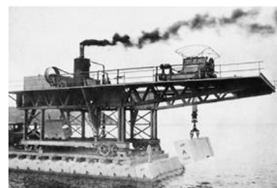
Fig. 1 Innovated machine (steam engine named Titan)-segment construction system for beak water at Otaru Horbor in 1890s: The first massive infrastructure of the modern Japan. (Photos from Hokkaido Agency Civil Engineering Department)
