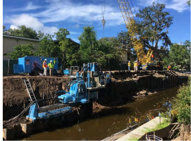
Fig. 6. Extraction of Old Sheet Piles (Left) and Installation of New Ones (Right)
