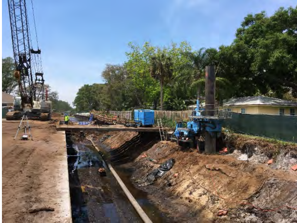
Fig. 5. Press-in Piling of Sheet Piles
