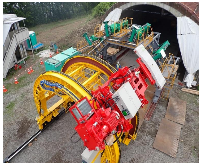
Photo 6. Erection machine for multi-divided precast lining
