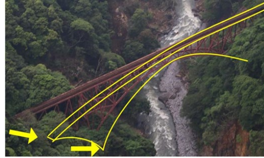
Fig. 2. Example of damage caused by the Kumamoto Earthquakes in 2016 (Minamiaso Area; assumed bridge deformation shown by yellow lines)
