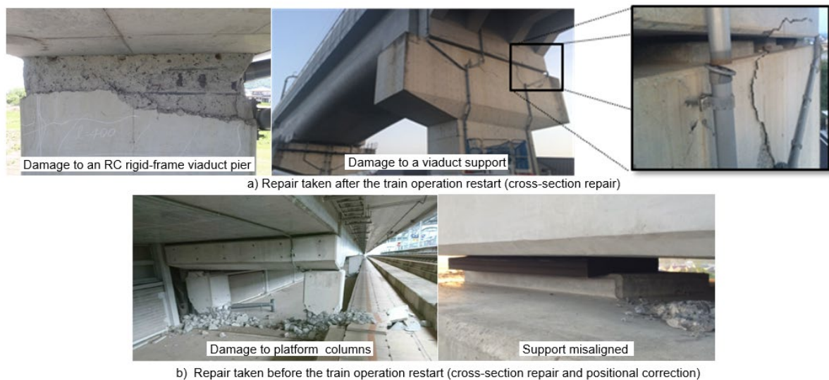
Fig.12. Technical support for the diagnosis of the Kyushu Shinkansen viaduct damaged by the Kumamoto Earthquakes in 2016
