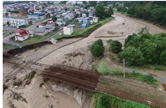
Fig. 4. Example of damage caused by Typhoon 10 in 2016 (river bridge)
