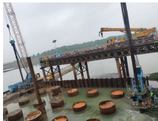
Fig. 5. Shortening of the construction period by using two press-in piling machines.
