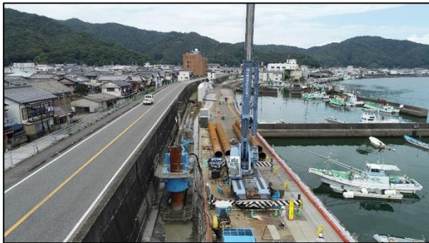
Photo 1. Pile Installation (Standard Gyropress Method)
