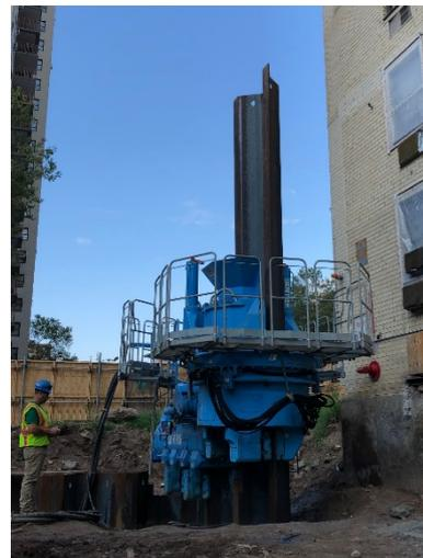
Fig.4. Sheet Pile Installation next to a High-rise Apartment Complex Site
