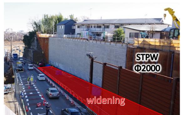
Fig. 1. Application of STPW (H=13m, lp=23m) for road widening projects. (Miyanohara et al.2018)
