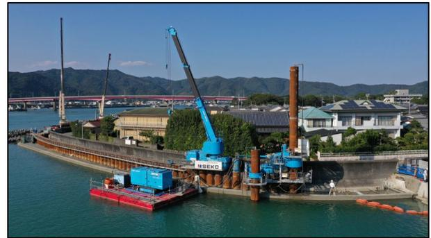
Photo 2. Pile Installation (Gyropress Method) with GRB Non-staging System)
