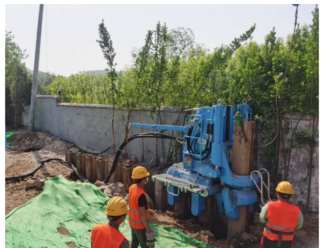
Fig. 4. Construction in proximity
