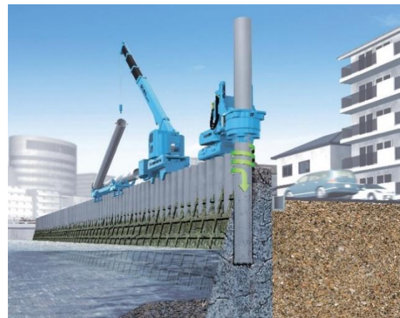
Figs. 8. Installation of Strut-free Piles for Construction of Robust Structure through Obstacles
