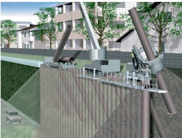
Figs. 8. Installation of Strut-free Piles for Construction of Robust Structure through Obstacles
