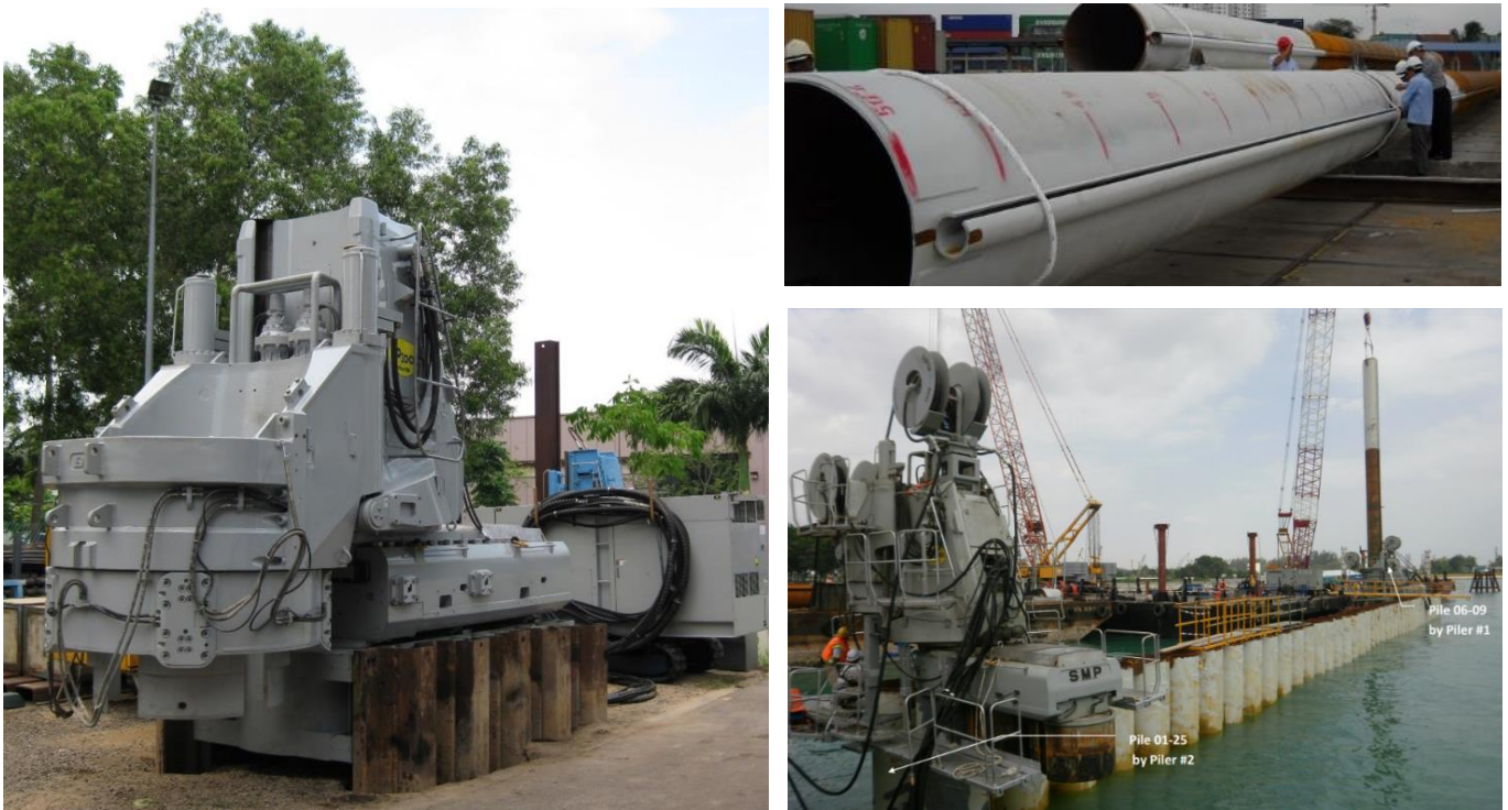
Figs. 6. GIKEN Kokan Piler & Tubular Sheet Piles
