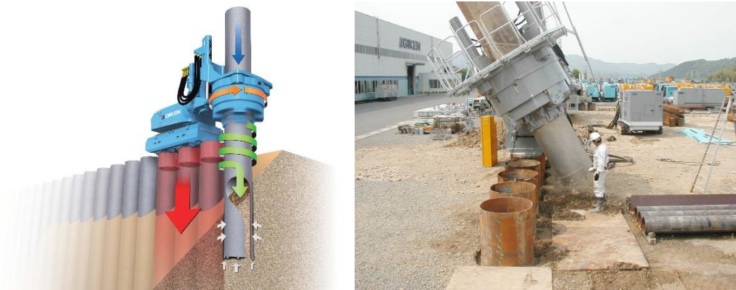
Figs. 10. The Gyropress Method
