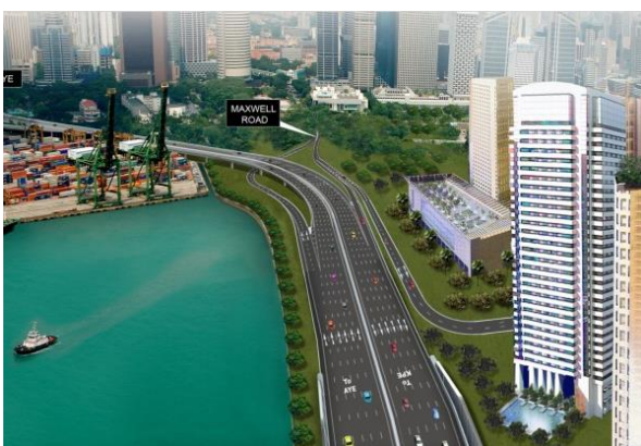
Fig. 3. Marina Coastal Expressway after Reclamation
