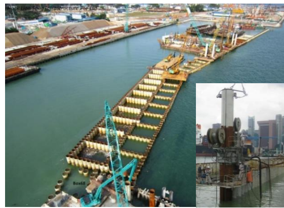
Fig. 4. Tubular Sheet Piles installed by Giken Kokan Piler
