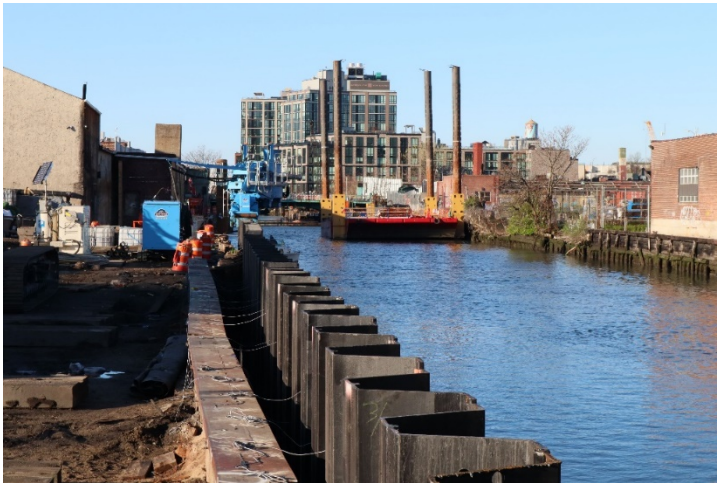
Fig. 4. Pressed-in Sheet Piles in the Gowanus Canal
