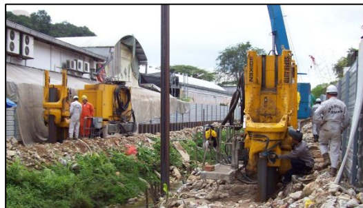
Picture 1 Installation of sheet piles in 2008
