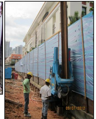
Picture 2 Installation of sheet piles in 2012
