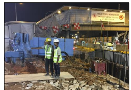
Picture 3 Press-in piling at a MRT site
