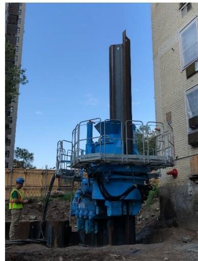
Fig.4. Sheet Pile Installation next to a High-rise Apartment Complex Site
