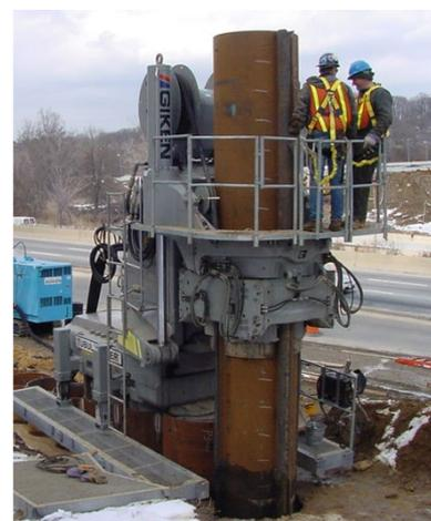
Fig.2. Tubular Pile Installation for Widening of Long Island Expressway
