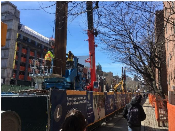
Fig.3. Press-in Piling Next to Sidewalk 83-89 Columbia Street Building #3 New Boiler Plant and Site Work
