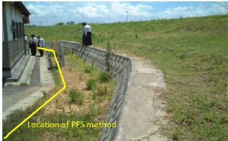
Photograph 1 After the PFS construction
