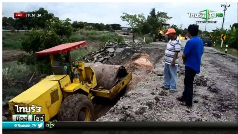
Photo 2 Restoration process of road settlement
