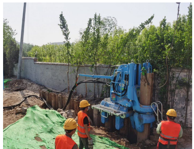
Fig. 4. Construction in proximity
