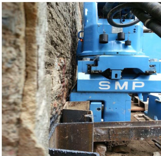
Figure 3 Zero clearance press-in method
