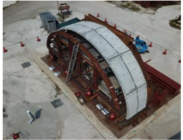
Photo 7. 2-ring assembled precast lining
