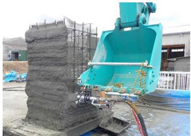
Photo 10. Direct print molding of buried formworks
