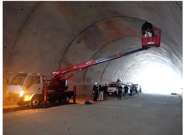
Photo 3. Verification test in the simulated tunnel
