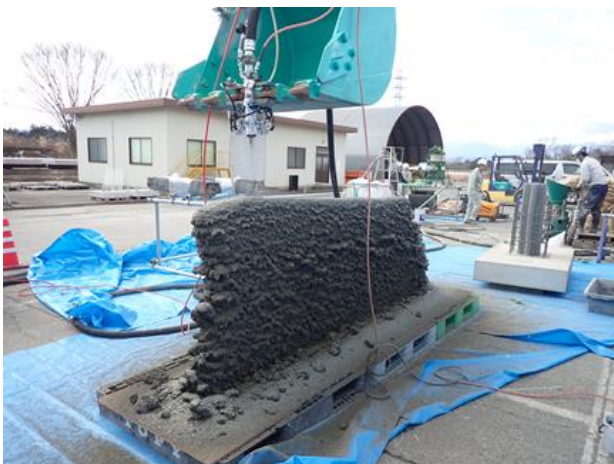
Photo 9. Direct print molding of a wall
