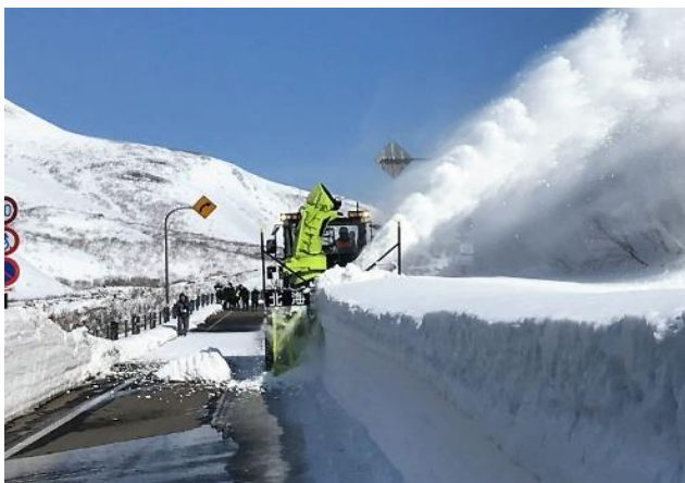
Photo 4. Automatic control of snow removal work
