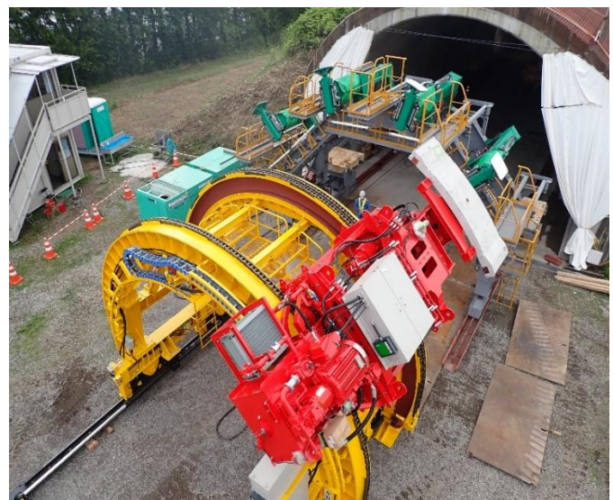
Photo 6. Erection machine for multi-divided precast lining
