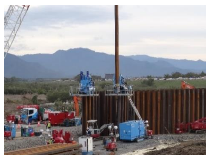
Photo 4 Construction of sheet pile wall by Silent Piler
