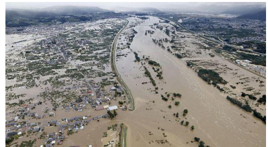
Photo 1 Torrential rain has caused rivers to flood along Chikuma River.
