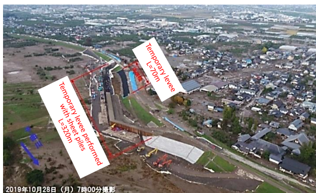
Photo2 Overview of Construction Site
