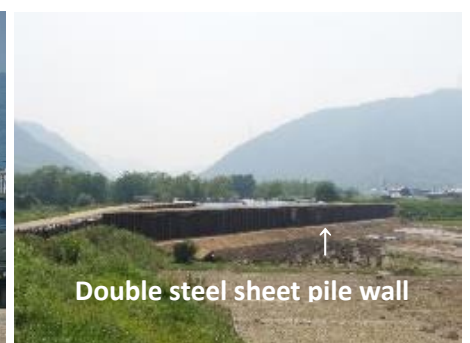
Photo 5 Tentative recovery work with steel sheet piles structure
