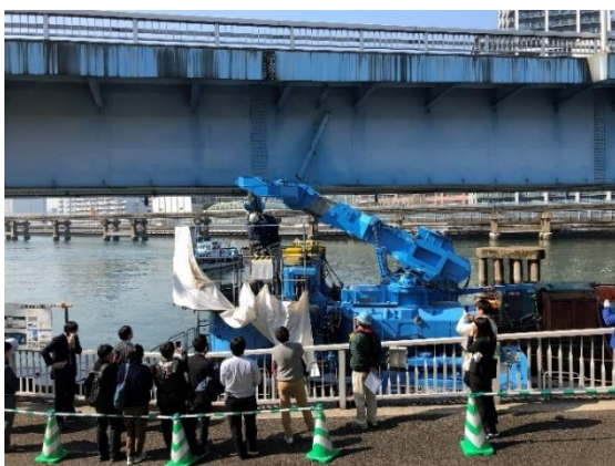
Photo 1. Overview of the piling construction
