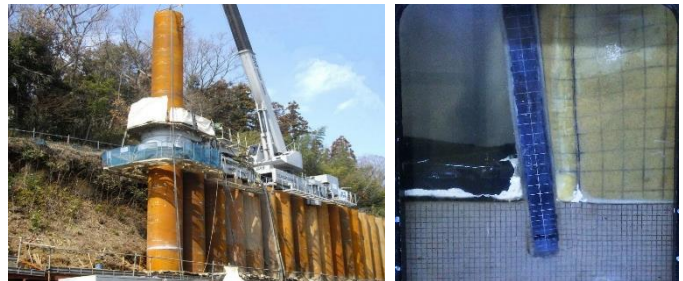
Tubular steel pile wall
