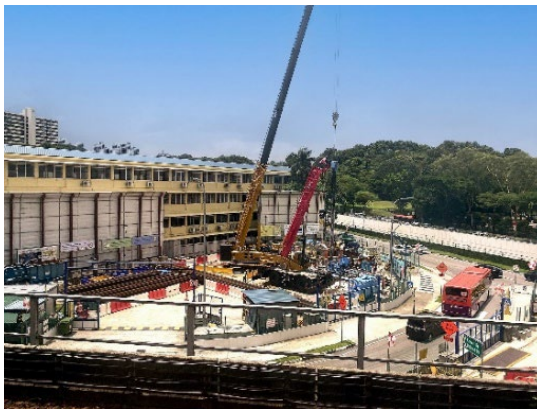
Fig. 4. Overview of the construction site (TS site)
