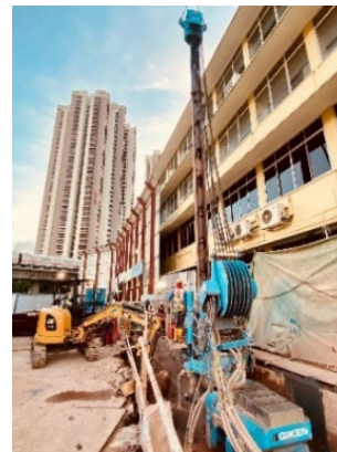
Fig. 5. Piling in progress (TS site)
