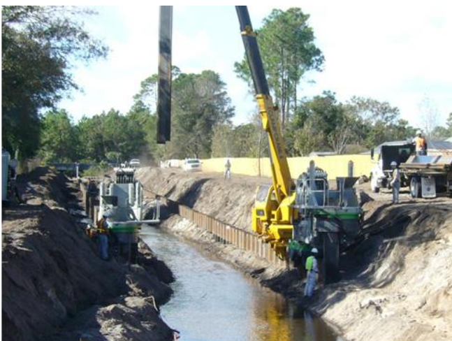
Fig. 11. Clamp Crane Pitching Sheet Piles to Silent Piler
