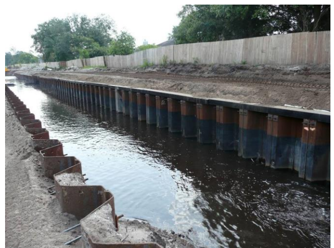
Fig. 12. Completed Sheet Pile Installation
