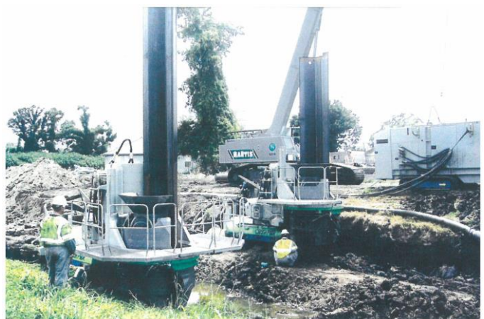
Fig. 5. Two Silent Pilers at Work
