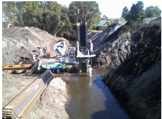
Fig. 10. Sheet Piles Installation for Weir
