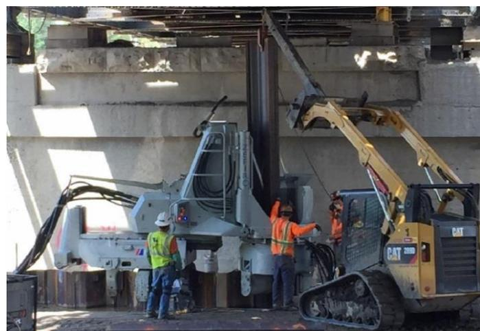
Fig. 5. A Short Section Being Placed on Top of the Lower Section for Splicing Under the Rail Girder
