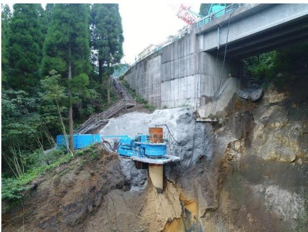
Fig. 7. Severe Erosion in Front of the Abutment
