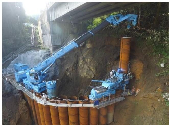
Fig. 13. Last Pile Supported by Clamp Crane during Splicing
