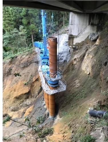
Fig. 11. Pile Installation on Heavily Eroded
