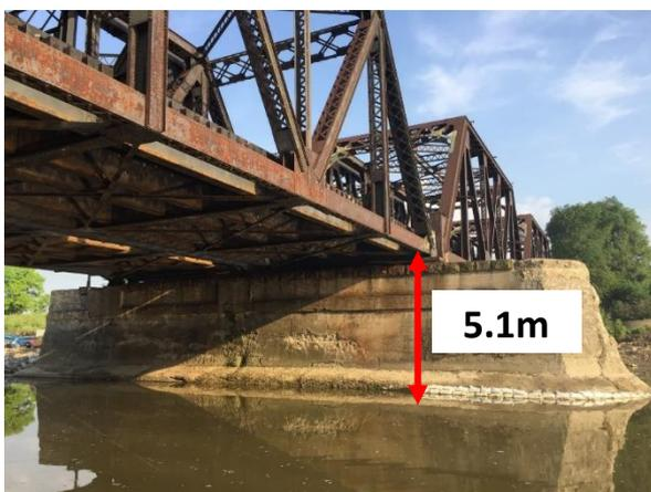
Fig. 1. Bridge Pier with Damaged Foundation
