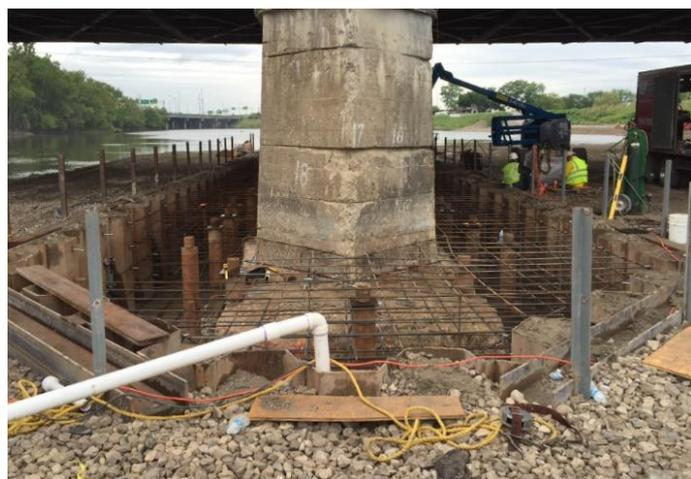
Fig. 6. Sheet Pile Cofferdam and Micropiles for Larger Encasement Footing
