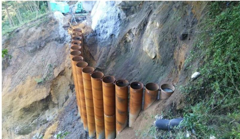
Fig. 14. Pile Installation Completed
