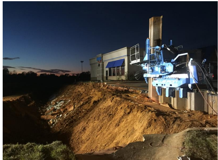
Fig. 11. Sheet Pile Installation during Night Time
