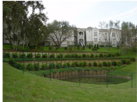
Fig. 6. Remediated and Landscaped Sinkhole
