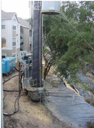
Fig. 5. Pipe Pile Being Pressed in at the Edge of Sinkhole
