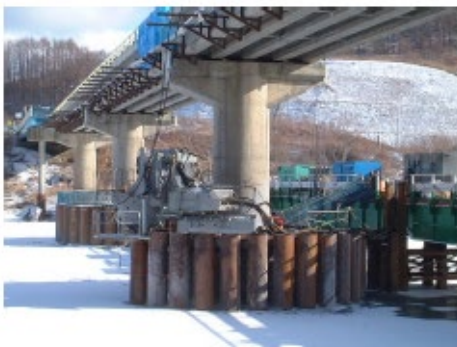
Photo 9. First installation in Hokkaido
