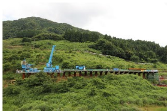
Photo 15 Construction in Nagasaki Prefecture
