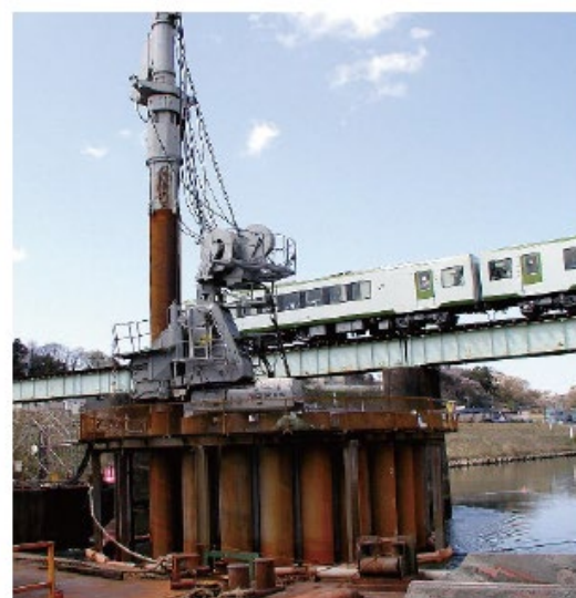
Photo 7. Construction in Ibaraki Prefecture with Tubular Piler for hard ground
