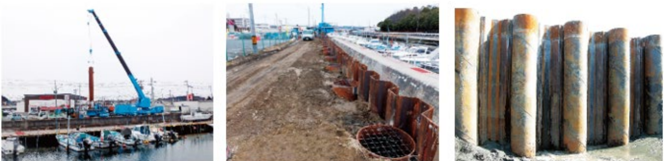
Photo 13. The construction site in Miyagi Prefecture with Combi-Gyro Method
