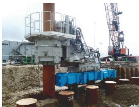
Photo 14 Construction in Iwate Prefecture
