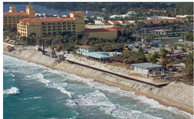
Fig. 3. Lantana Emergency Seawall Construction with Pressed-in Sheet Piles
