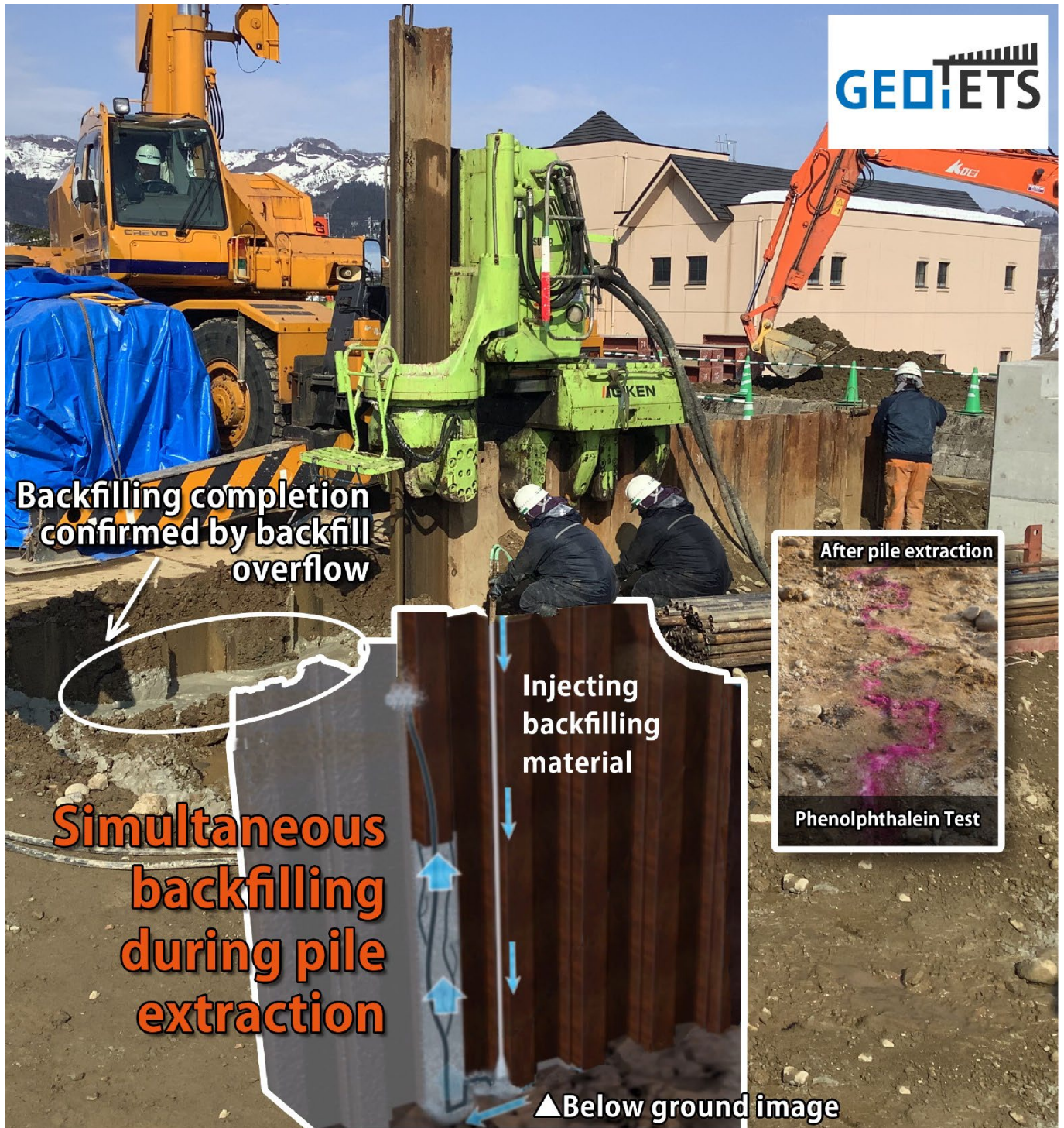
Fig. 1 Overview of GEOTETS Method
