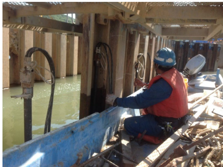
Fig. 4. Backfilling (above water)
