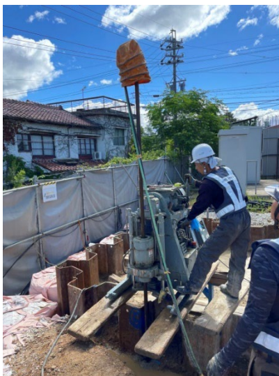
Fig. 3. Insertion of injection pipe
