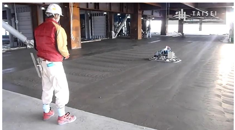
Fig. 10. Automatic concrete slab finisher
