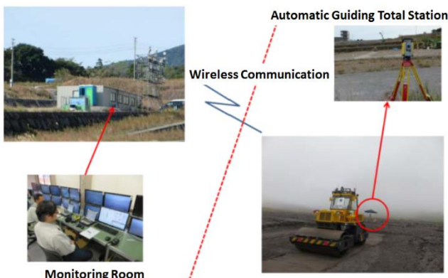
Fig. 7. Verification test of autonomous unmanned vibration roller
