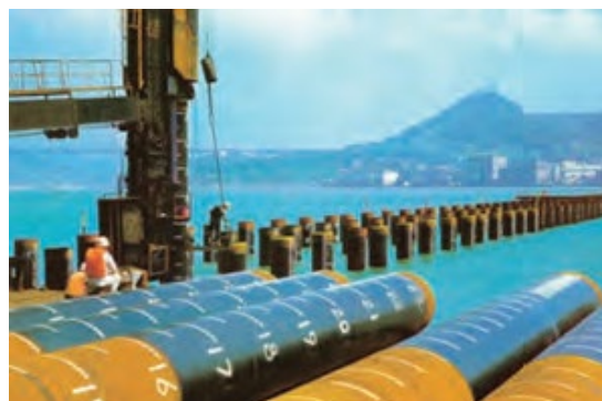
Photo 2 Heavy-duty anticorrosion steel pipe pile with polyethylene coating (Black part is the covering material)
