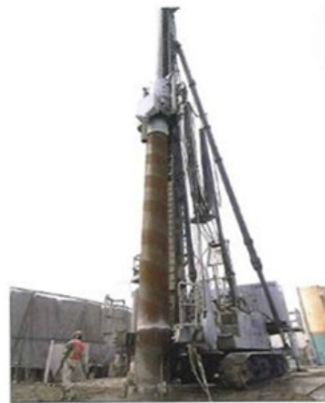
Photo 7 Steel Pipe Soil Cement Piler 15)
