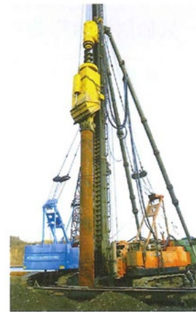
Photo 5 3-point support pile driver rig 15)
