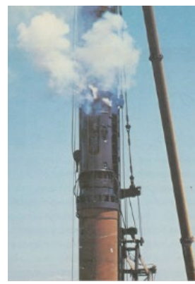
(c) Diesel hammer 9)
