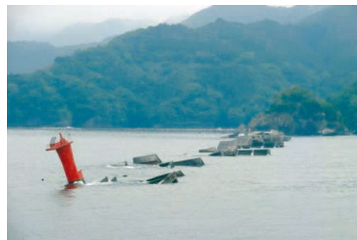
Photo 1.10 Damage to Kamaishi Bay mouth breakwater 10)
