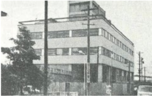
Photo 1.1 Niigata Telecommunications Dept. Office Building 1)
