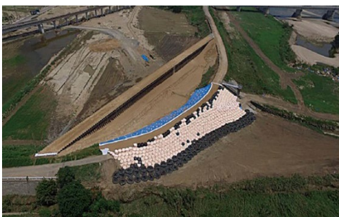
Photo 2.3 Double cofferdam of steel sheet piles driven 24 hours a day 18)
