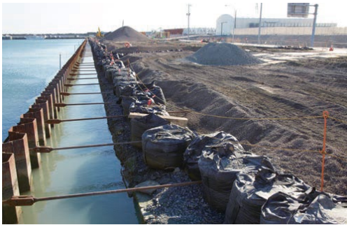
Photo 1.11 New Installation of steel sheet piles of designed water depth - 7m quay 13)
