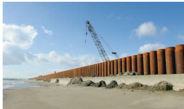
Photo 1.12 Installation of tubular sheet piles on the Higashihama coastal embankment of Ishinomaki Port 14)
