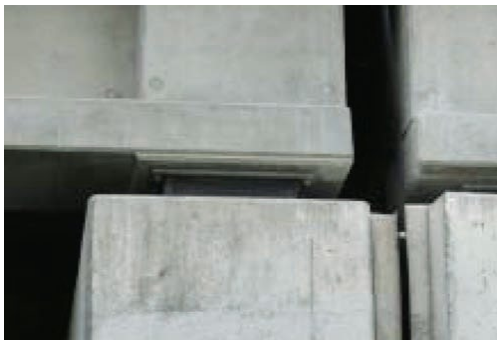
Photo 1.9 Bearing deformation 11)
