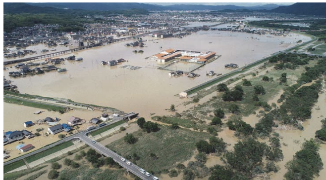
Photo 2.2 Collapsed Odagawa embankment 18)
