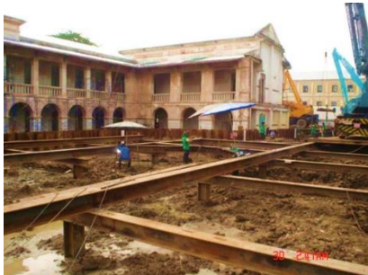
Photo 2 Sheet pile was driven around existing palace
