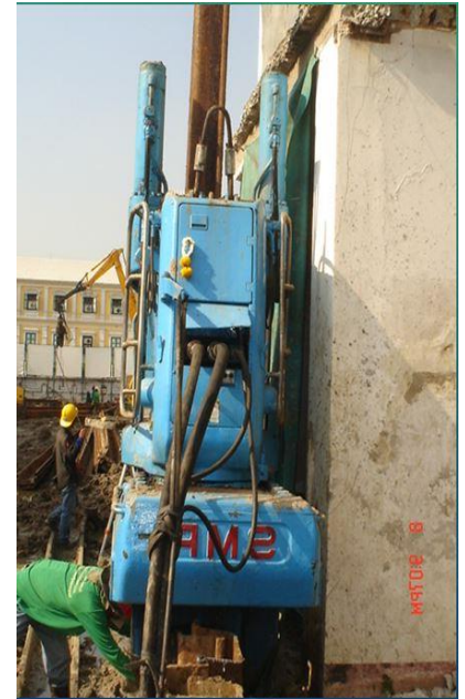
Photo 4 Silent Piler (AT90 model) and existing of Saranrom palace wall
