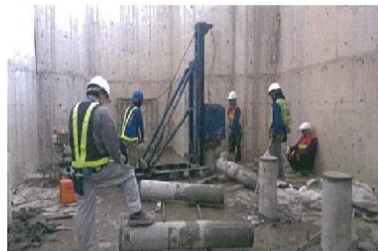
Photo 6. Piling work of micro spun pile
