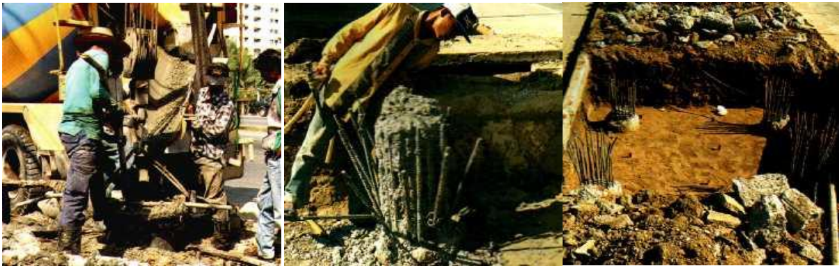
Photo 4. The schematic technique of dry process bored pile
