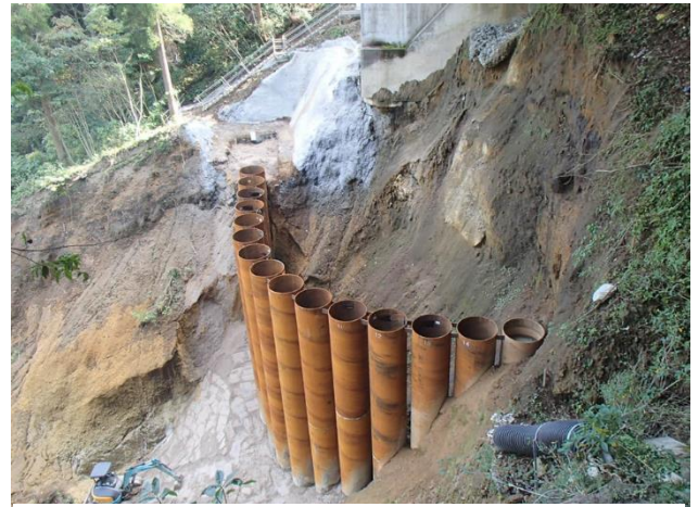
Photo 3 A view of after Press-in operation
