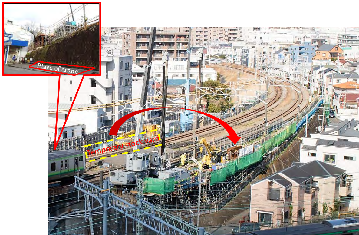
Picture5 carry-in the equipment
