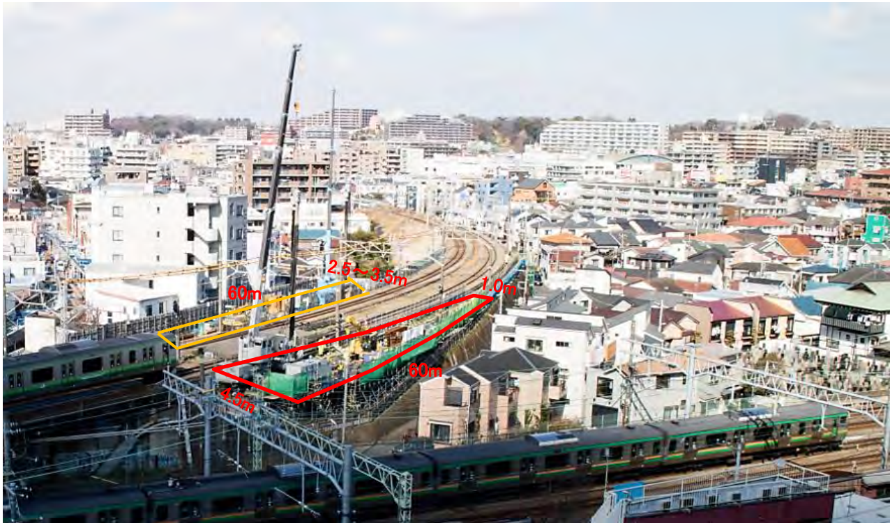
Picture1: Construction overview
