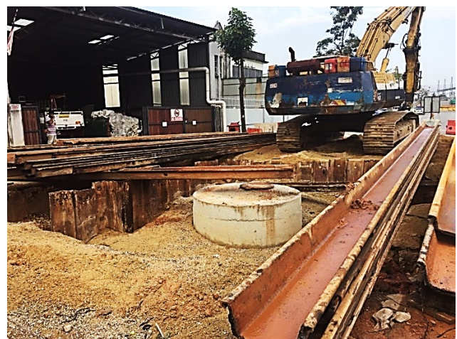
Fig. 2. Sheet pile work on construction site
