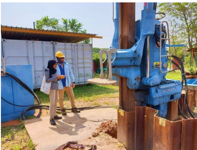
Fig. 5. Operating the Standard Press-In machine for the first time
