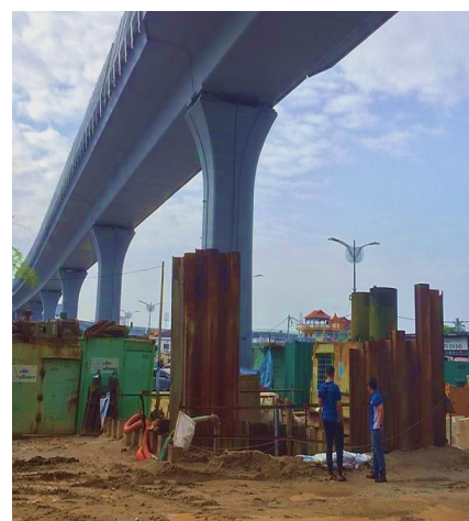
Fig. 4. Sheet pile installation under MRT Line
