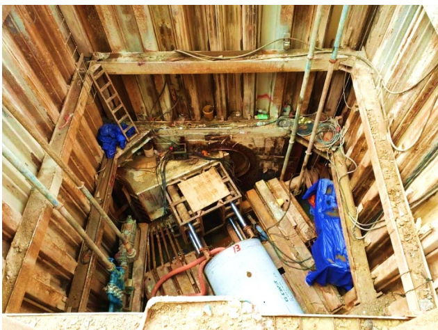
Fig. 3. A braced cut excavation by using a sheet pile
