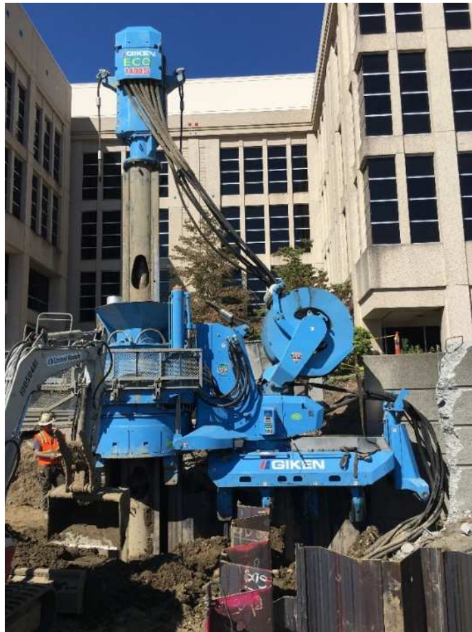
Fig. 3. Press-in piling with auger attachment (Photo: Blue Iron Foundations and Shoring LLC)
