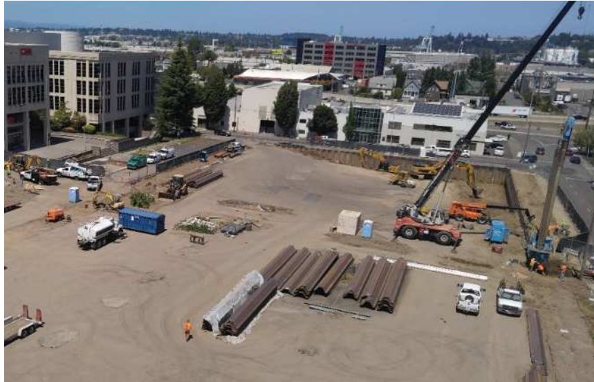
Fig. 4. Press-in piling (far right) followed by excavation (Photo: Blue Iron Foundations and Shoring LLC)
