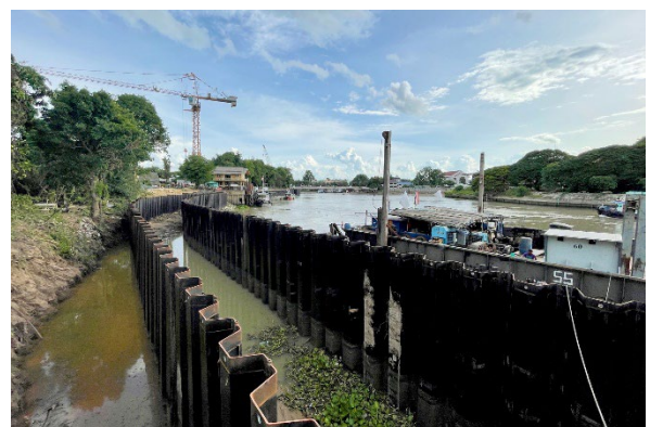
Fig. 4. Double hat-type sheet pile wall
