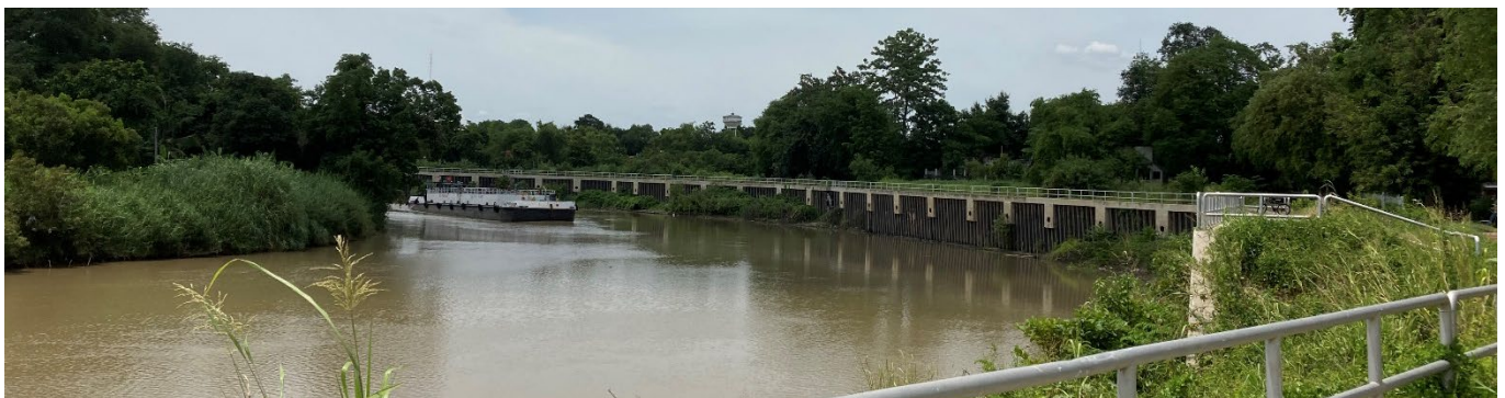
Fig. 2. U-shaped sheet pile revetment in Phase 1
