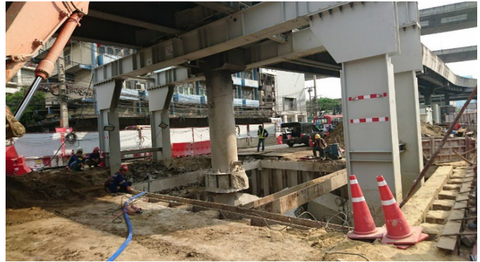
Fig. 6. Site condition after sheet pile installation
