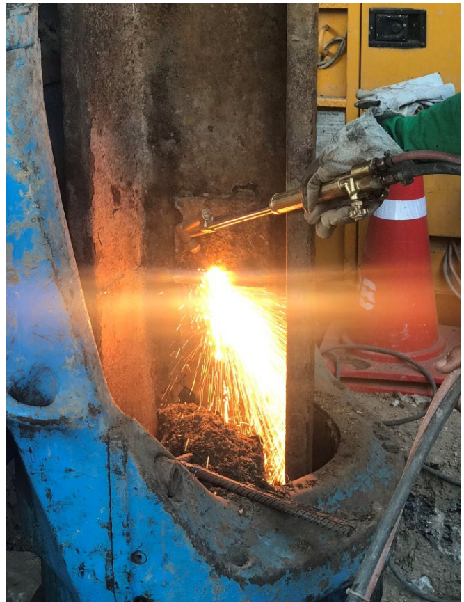
Fig. 8. Sheet pile connection
