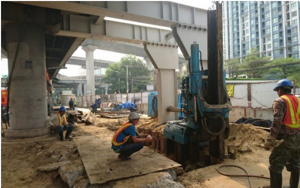
Fig. 5. Sheet pile installation at Chainage 28+200
