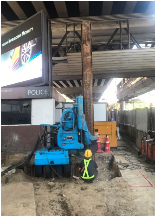
Fig. 7. Sheet pile installation at Chainage 29+300
