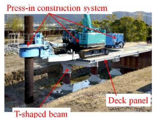
Fig. 2. Press-in construction system for the Implant Bell Cap Bridge
