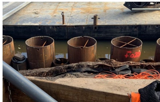
Fig. 4. 23m deep x 508mm diameter piles with shorter small diameter closure piles between
