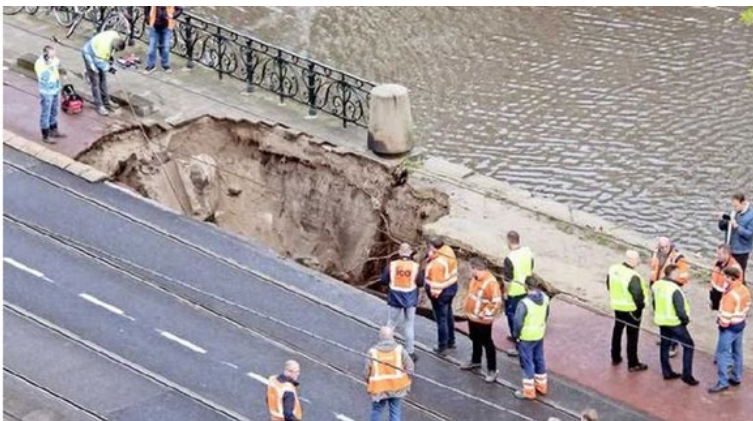
Fig. 1. Photograph of sink hole appearing alongside the canal wall (Giken, 2023)
