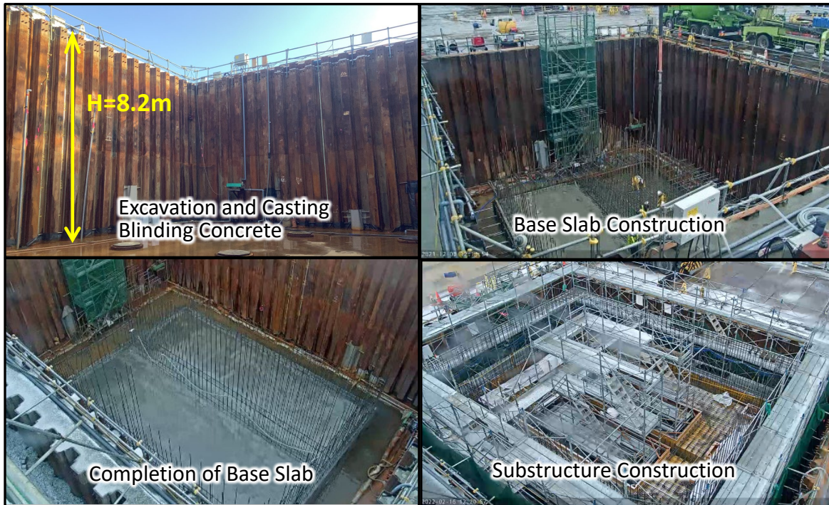
Fig. 6. Excavation and Construction of Substructure
