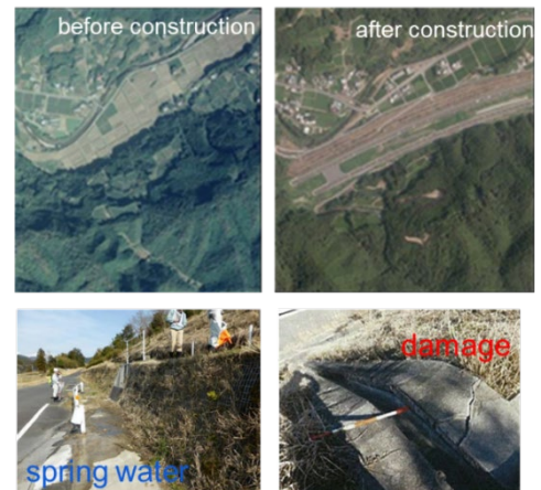
Photo 2 Target embankment with damage
