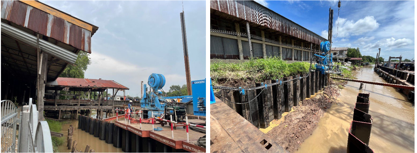
Fig. 10. Construction performed adjacent to buildings
