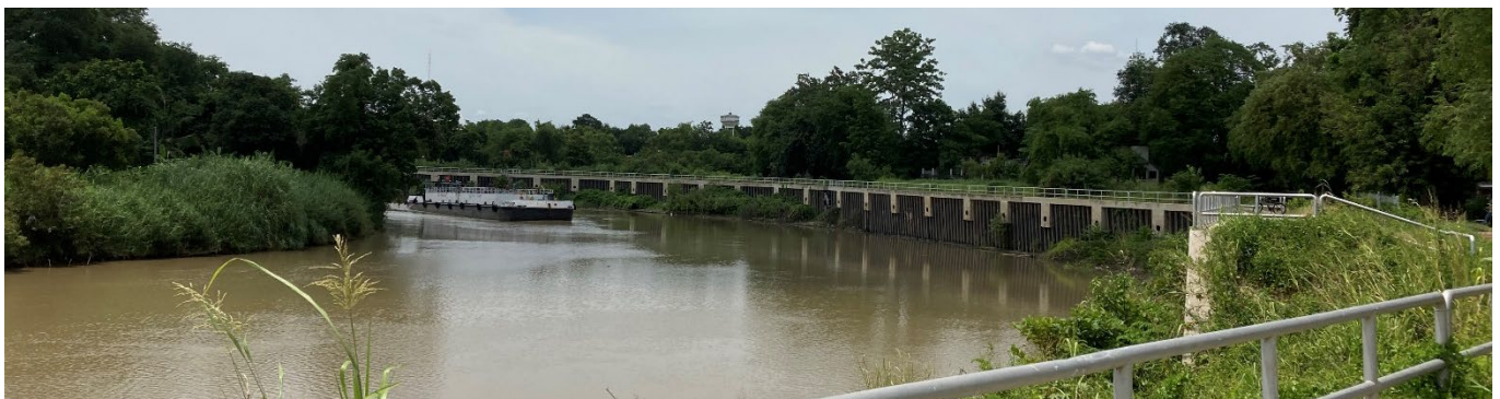
Fig. 2. U-shaped sheet pile revetment in Phase 1
