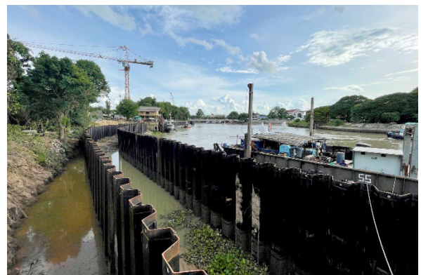
Fig. 4. Double hat-type sheet pile wall
