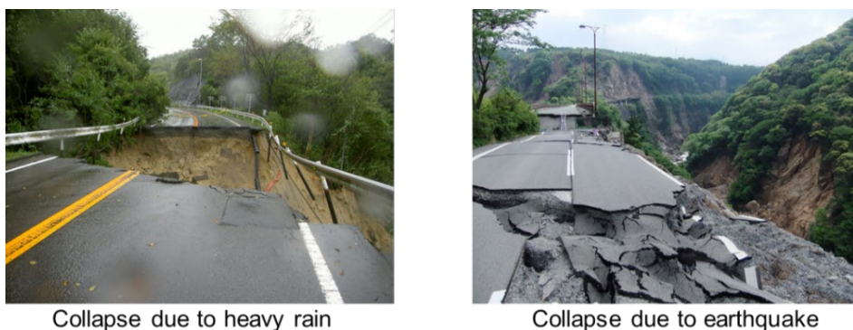
Fig. 1. Collapses of road embankment due to heavy rain or earthquake
